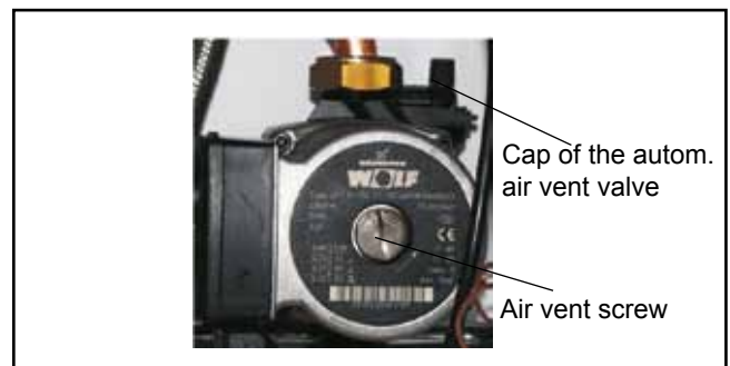
Fig.: Automatic air vent valve on the heating circuit pump
