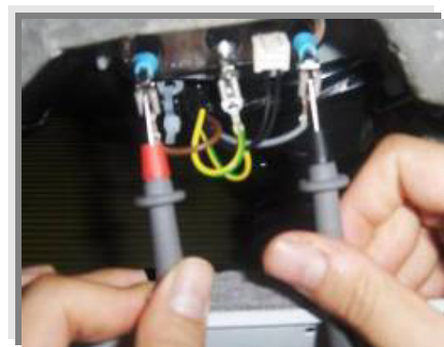
Figure 12. Checking the component
